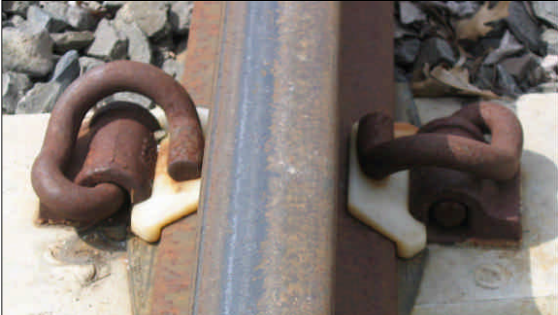
Figure 15 – Example fastening system on non-plated concrete turnout ties
