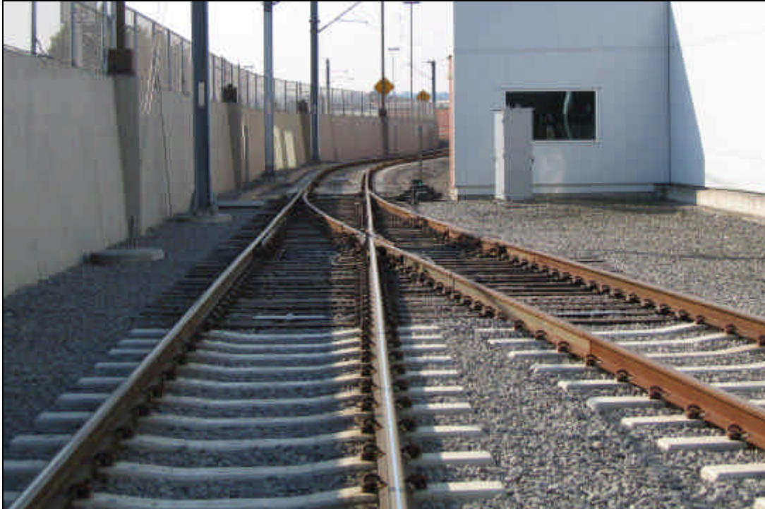
Figure 1 – Wood turnout ties within standard concrete tie track
