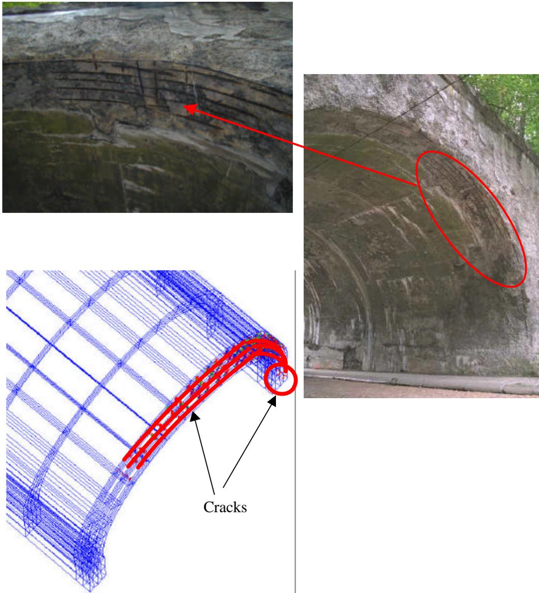
Figure 10- Arch Barrel Spandrel Wall Separation and Longitudinal Cracks in the Arch barrel
