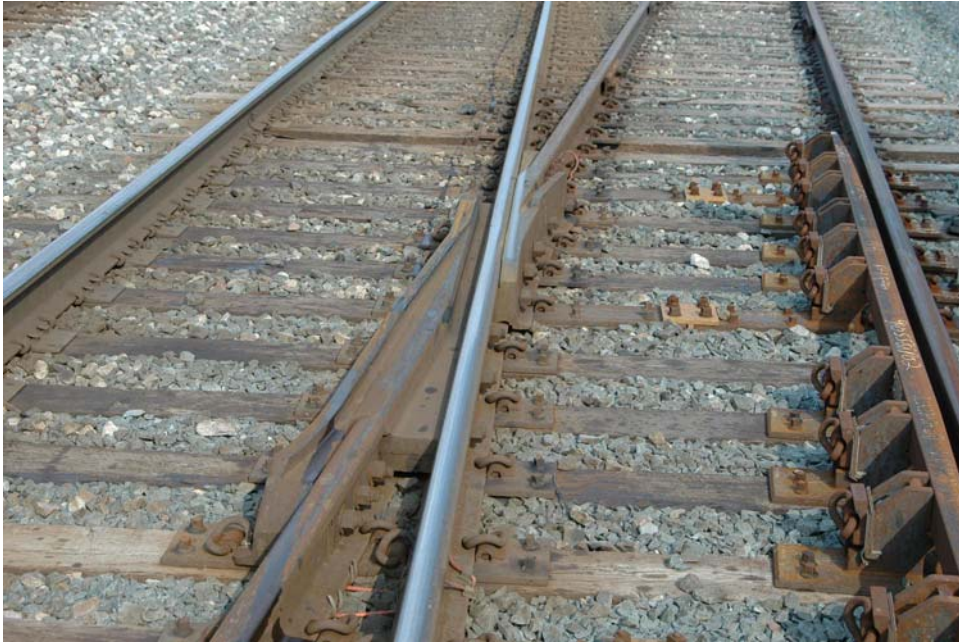
Figure 14. Typical Lift Frog Following Installation, Tracy, Indiana.
