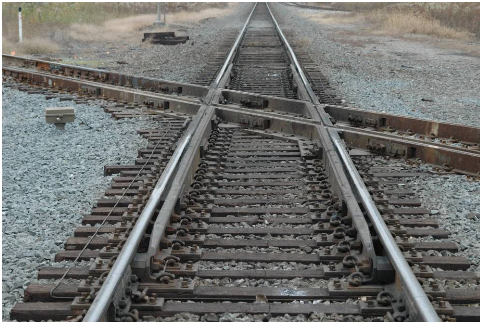
Figure 4. Shelby FBF Following Installation
