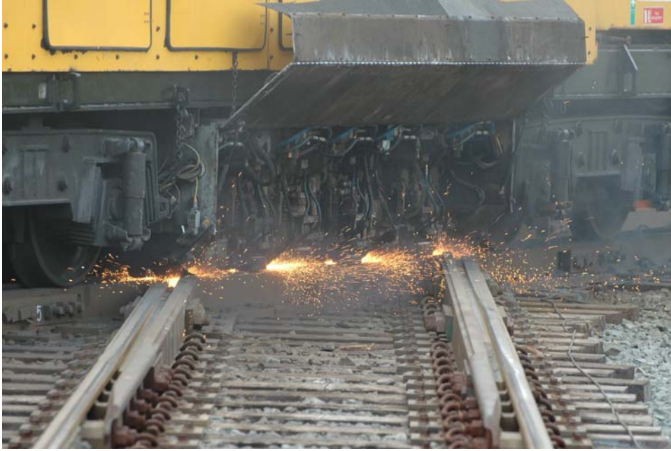
Figure 11. Shelby Flange Bearing Diamond During Grinding
