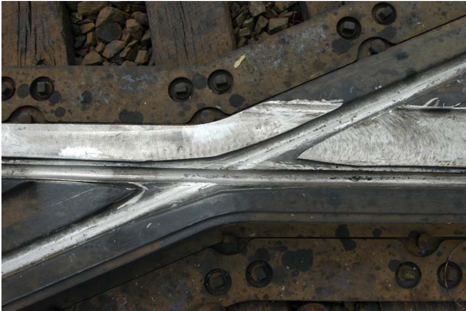
Figure 12. Shelby Flange Bearing Diamond Following Grinding
