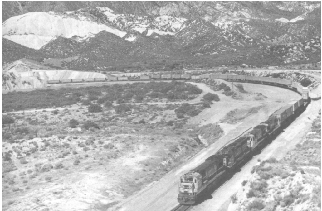
Figure 6-9 Heavy Curvature on the Santa Fe - Railway Technical Manual – Courtesy of BNSF
