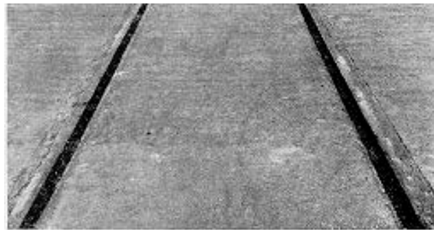
A Flangeway Installation
